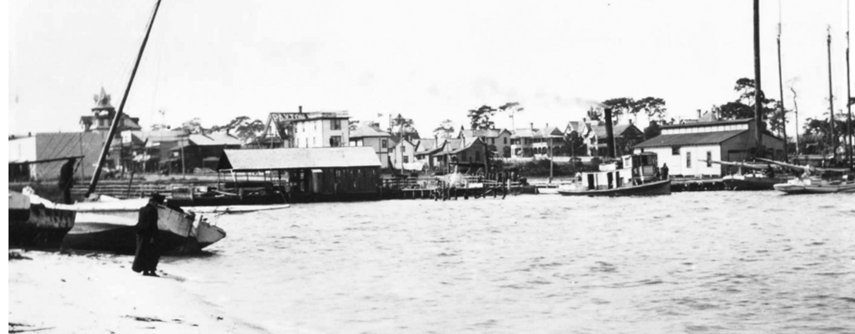
Waterfront at the turn of the century: City fathers' vision included open parks, with a yacht club, and not the hodgepodge of buildings, commercial wharfs and derelict boats. The power plant, right, was built in 1899 over the water at the site of SPYC's present parking garage. A plaque in the sidewalk on Central Avenue commemorates this historical fact. CITY OF ST. PETERSBURG
